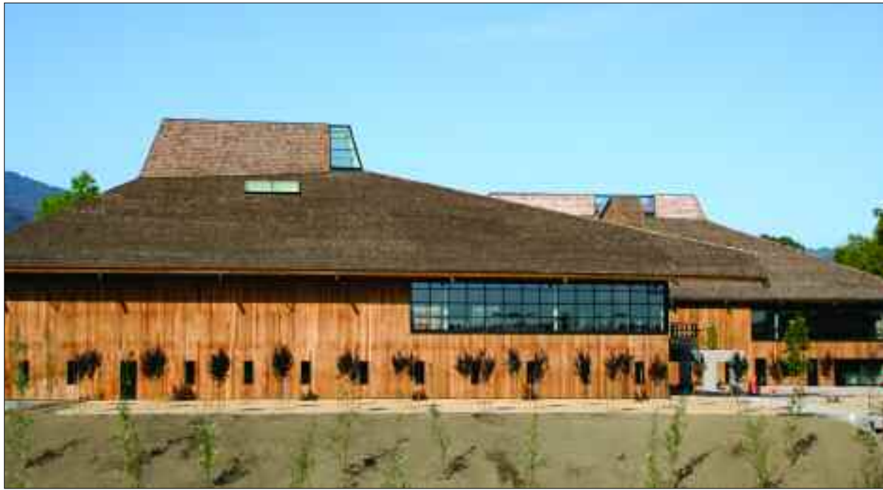
Foothill Is Turning 50! Join us as Foothill College kicks off its 50 th anniversary celebration with the grand opening of the new Foothill Campus Center (above, below) and Lower Campus Complex Tuesday, Sept. 25, from 4 to 7 p.m. For details, access www.foothill.edu/50 .
